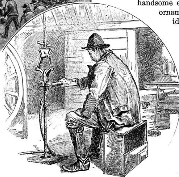
DRILLING IN THE DERRICK-HOUSE (PENNSYLVANIA OIL REGION).
